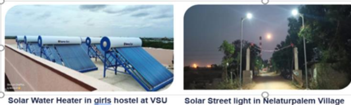
Solar Water Heater in girls hostel at VSU
