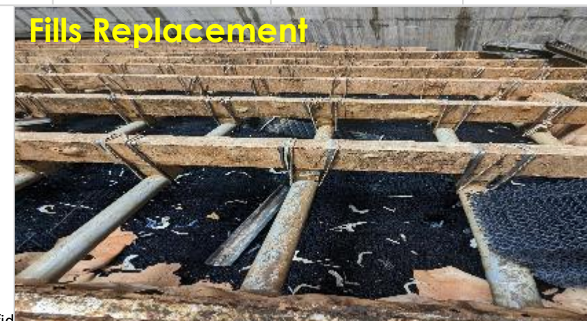
New Fills, Nozzles fixed
